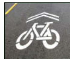
Shared Lane Marking
